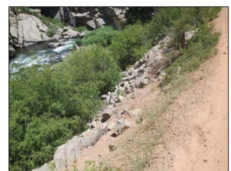
Photo 4 Steep Slope to River
