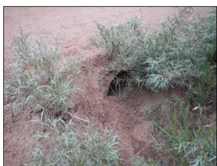
Photo 1 Culvert Blocked with Sediment
