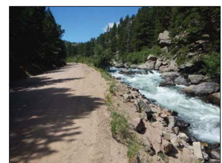
Photo 3 Steep Slope to River
