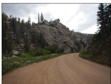
Photo 1 Typical Cut Slope Near Curve
