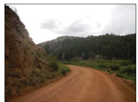
Photo 5 Typical Rock Cut Near Curve
