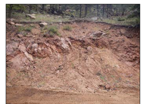
Photo 3 Typical Cut Slope
