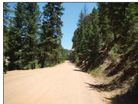
Photo 2 Wider Roadway Section
