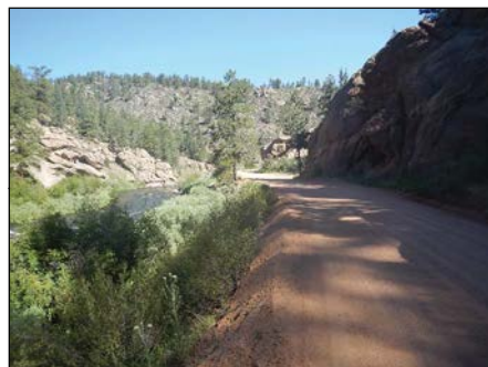
Photo 3 Typical Road Shoulder Drop
