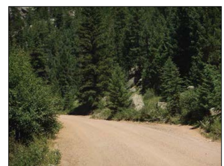
Photo 4 Typical Roadway Section
