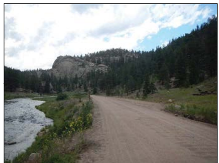
Photo 3 Typical Washboard Surface
