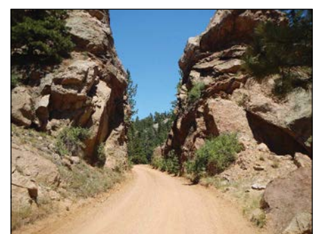
Photo 5 Large Rock Cut near Curve
