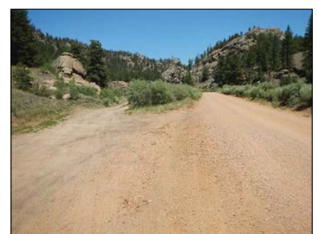
Photo 5 Approach to Road Intersection
