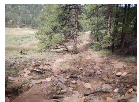
Photo 5 Drainage with Erosion
