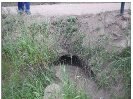
Photo 5 Culvert Blocked with Sediment
