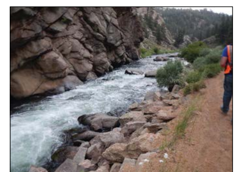
Photo 2 Banks Too Steep to Support Vegetation
