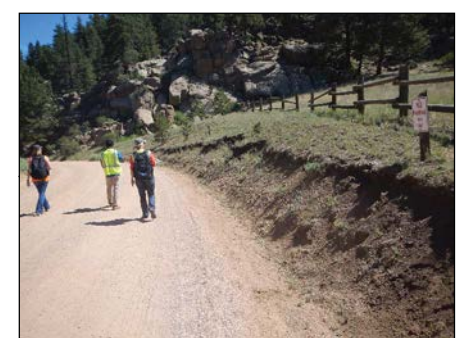
Photo 3 Cut Slope Near Campground
