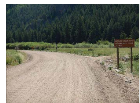
Photo 2 Typical Roadway Section
