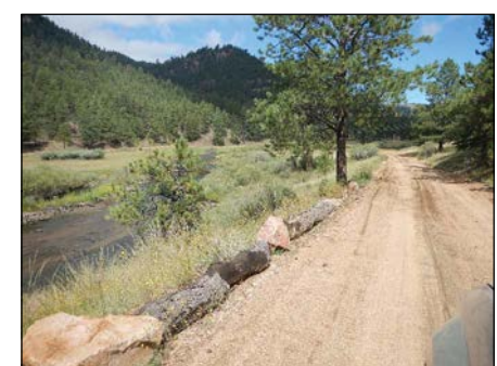
Photo 2 Roadside Erosion Protection
