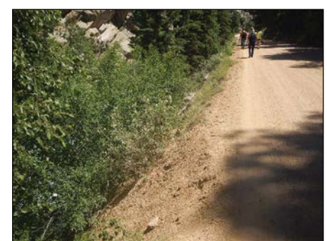
Photo 4 Steep Slope to River
