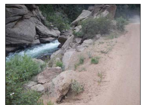
Photo 4 Limited Vegetation on Slope
