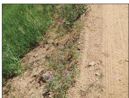
Photo 1 Shoulder with Loose Sediment
