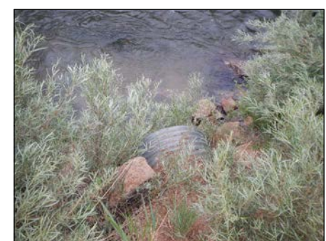
Photo 2 Culvert Outlet to River
