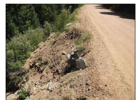
Photo 2 Culvert Outlet
