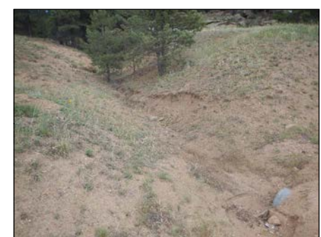
Photo 2 Hillside Drainage Erosion
