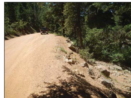
Photo 4 Limited Vegetation on Slope
