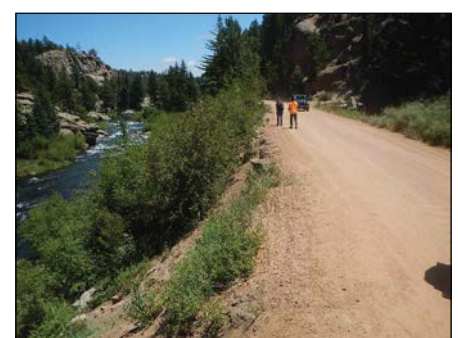
Photo 5 Steep Slope to River
