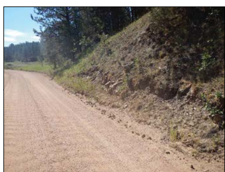
Photo 1 Typical Cut Slope
