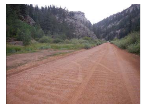
Photo 2 Typical Washboard Surface
