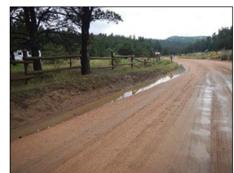
Photo 2 Roadway Drainage
