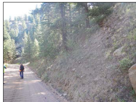
Photo 4 Typical Loose Cut Slope
