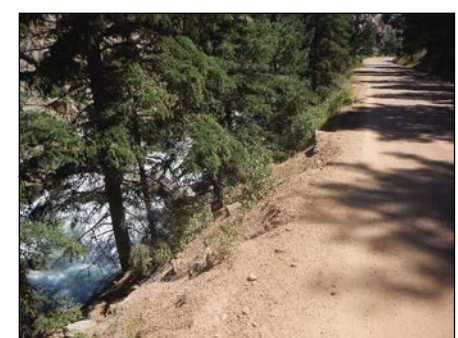
Photo 3 Limited Vegetation on Slope
