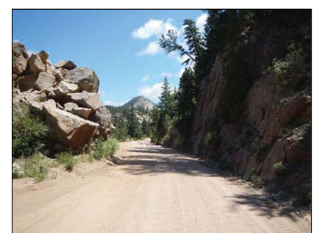
Photo 4 Narrow Rock Cut Section
