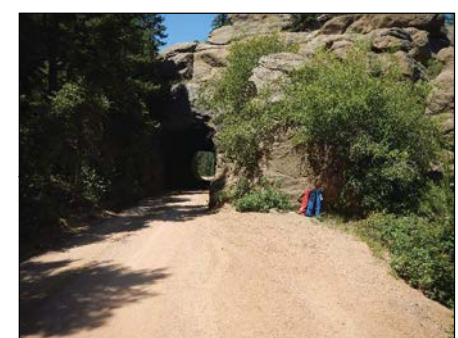
Photo 3 Approach to Tunnel, Pullout
