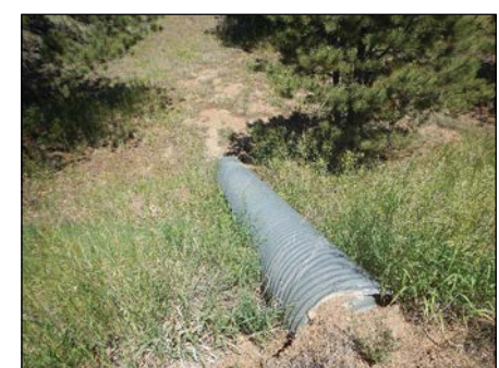
Photo 2 Culvert Rundown
