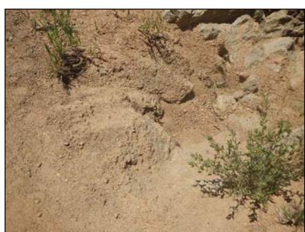
Photo 1 Culvert Blocked with Sediment
