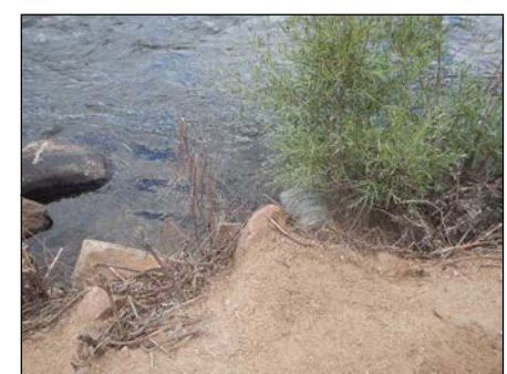
Photo 3 Culvert Outlet to River
