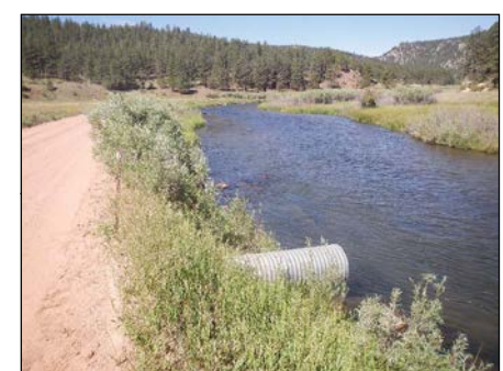
Photo 3 Culvert Outlet to River
