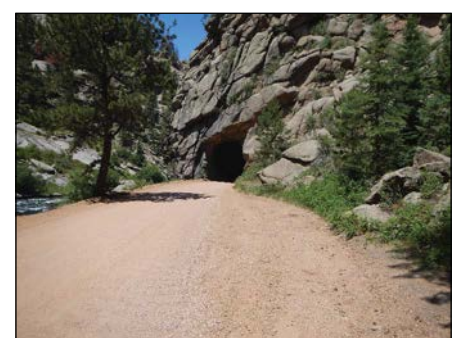
Photo 5 Typical Wider Roadway Section
